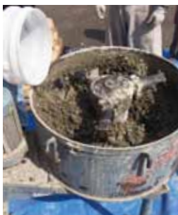
▲ 裏込め材練り混ぜ
