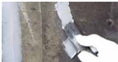
Sealing along crack edges
