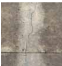
Cleaning of surface
